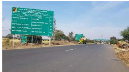
Sign boards at Toll plaza
