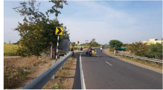
Km. 29+900 Crash barrier at bridge section
