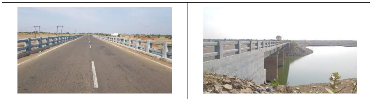
Figure 4.1: Overall view of the major bridge at Km 21+878
